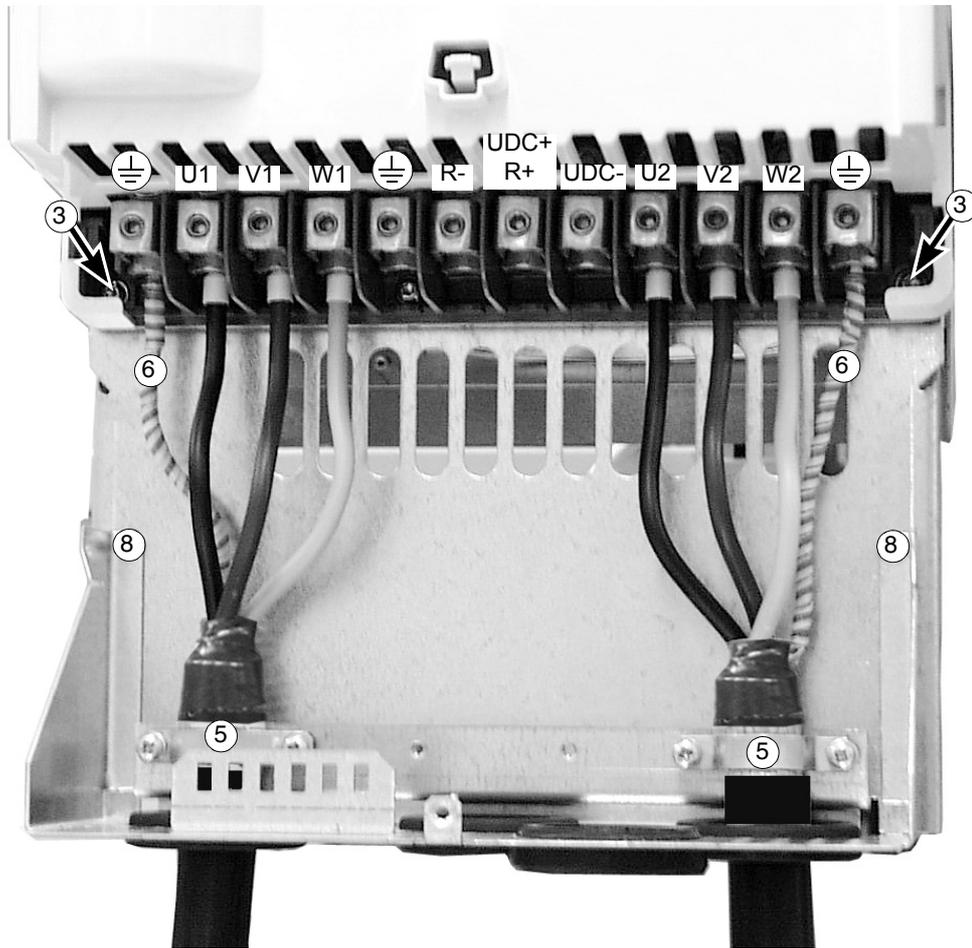
Frame size R6: Cable lug installation [16 to 70 mm<sup>2</sup> (6 to 2/0 AWG) cables]
